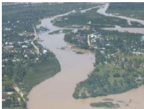
An aerial view of the damages caused by Cyclone Indlala
