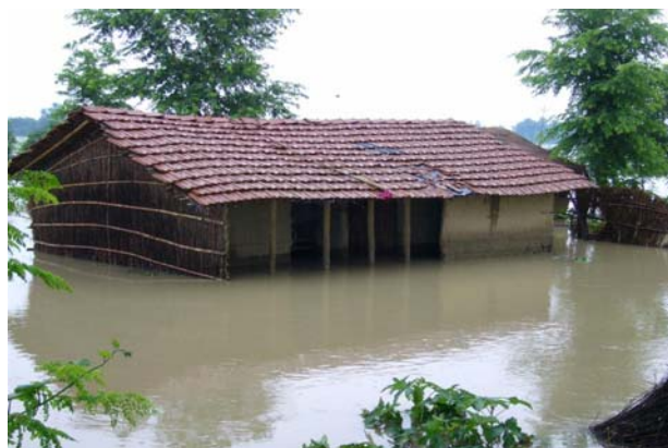
Flooded house in Dhanusa district, Central Terai. Federation
