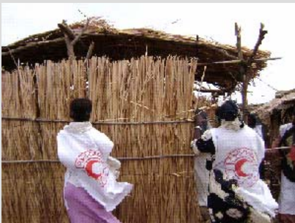
Sudanese Red Crescent volunteers constructing an emergency shelter in Gezira State.
