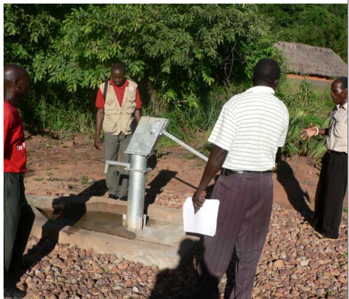
Zambia Red Cross staff and volunteers and the beneficiaries inspecting a rehabilitated water point (borehole) in Luangwa District ( Zambia Red Cross )
