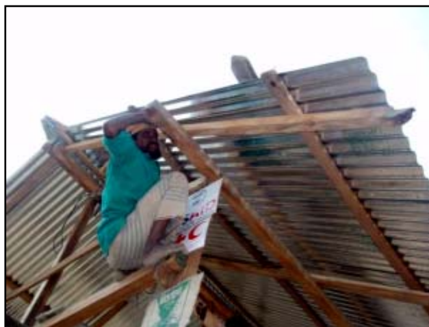
A shelter test case being constructed in Bagerhat.
