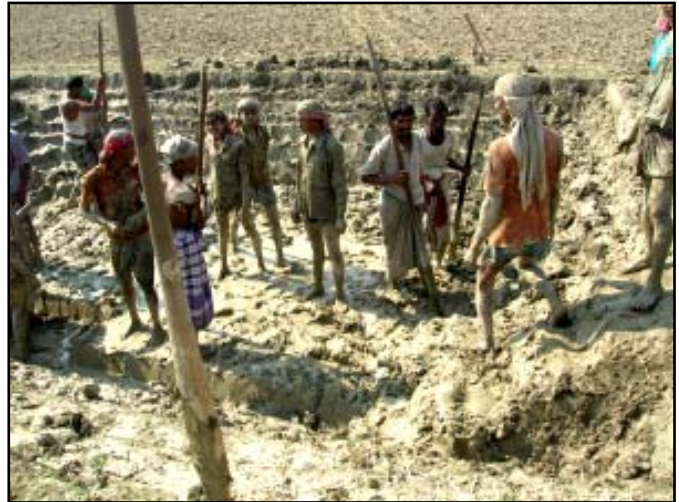
Digging the pond to build the mud plinth at Bagerhat district.
