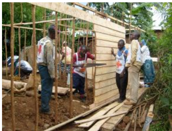
Volunteers built houses with wooden materials to accommodate victims
