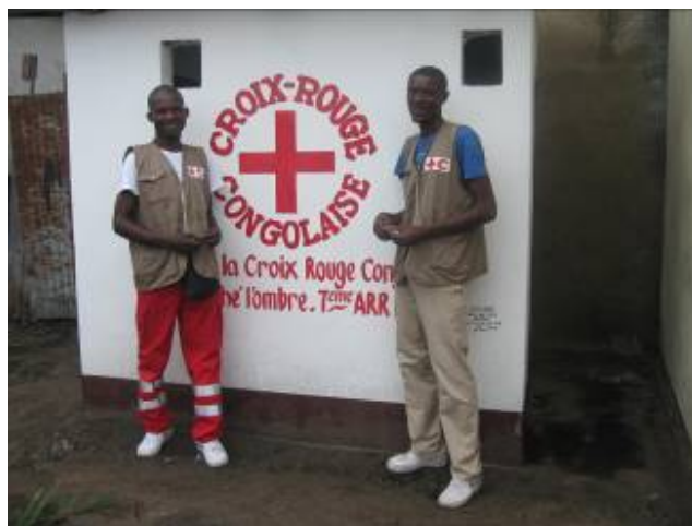
A latrine built by the Federation RDRT-WATSAN members in Brazzaville
