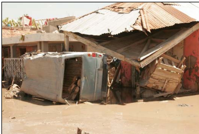
The hurricanes hit the country hard: houses were completely destroyed Source: International Federation
