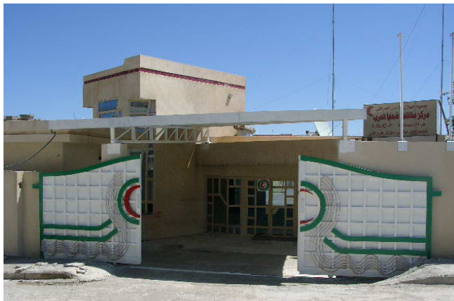
The construction of the Suleymaniah branch's fence and information-guard house was finalised by the end of March 2009.
