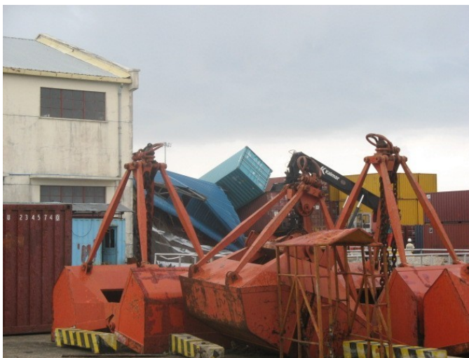
The main port in Yangon that is due to be out of action for up to three weeks.
