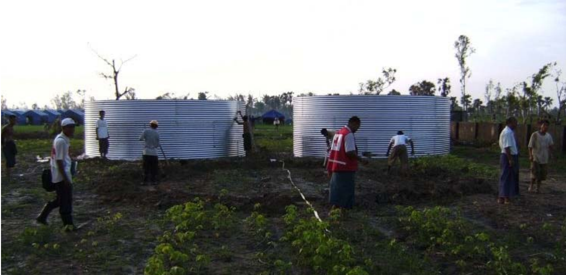
Water and sanitation tanks go up in Labutta. (International Federation)
