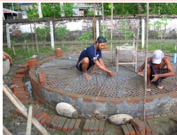
Significant capacity in water, sanitation and hygiene promotion continues to be built within the Myanmar Red Cross Society, thanks to the extensive support established by the Nargis Operation's water, sanitation and hygiene promotion programme. In this picture, a Ferro cement tank with a 22,500-litre capacity, is being constructed in Bogale township. (Photo: Zaw Oo / Myanmar Red Cross Society)
