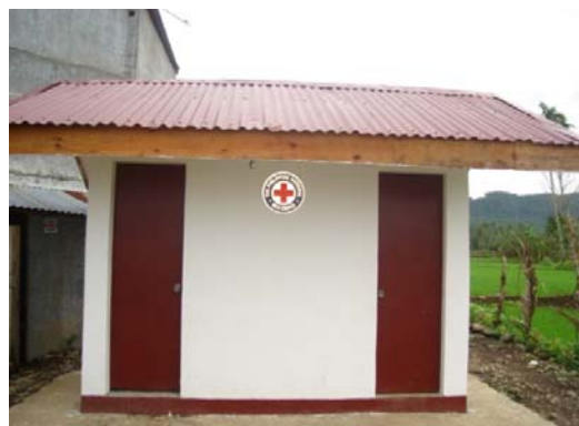
One of the latrines that were constructed in the evacuation camp to cater to the needs of the evacuees (International Federation)
