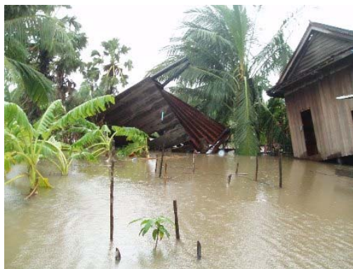
One of the numerous houses destroyed by Typhoon Ketsana in Cambodia: Over 1,780 homes have been flooded, destroyed or seriously damaged in the aftermath of the typhoon. (Photo: Sinal Peanh, Minority Organization for Development and Economy/ED)
