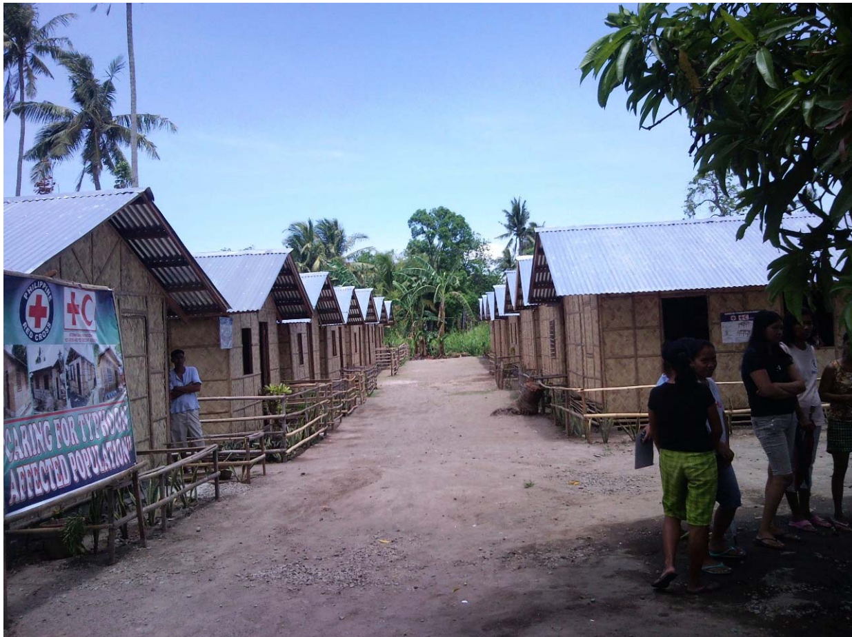
Significant progress has been made in ensuring that typhoon-affected families have a roof over their heads. As of April, some 210 transitional shelters, with latrines and septic tanks, had been completed [including those pictured above, in Laguna], with construction of 2,000 others in planning or in progress. However, to date, only 1,900 transitional shelters [of the 6,500 planned] and 4,500 shelter repair kits [of the 10,000 planned] have been resourced. Shelter activities remain significantly under-funded; additional support from partners is needed. (Photo: Alexander Mikadze/IFRC)
