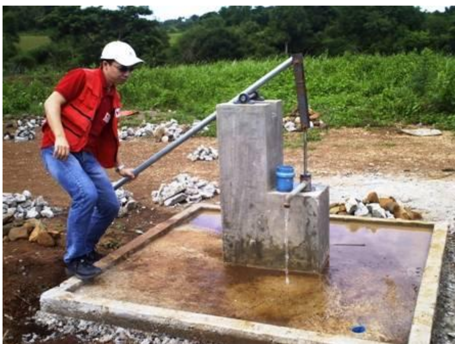
An IFRC delegate tests a hand pump of one of the seven boreholes sunk at Antipolo, Rizal. (Photo: Alexander Mikadze/IFRC)
