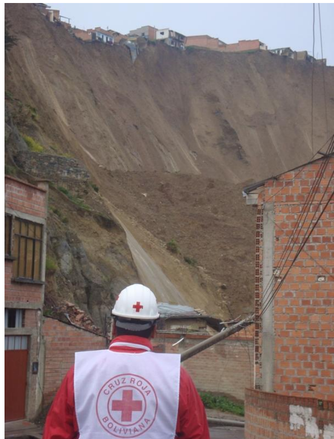
Some 800 homes were destroyed when a hillside collapsed in Kupini, a neighbourhood in the capital city of La Paz. Source: BRC
