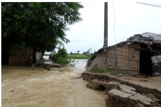
Flood water entering the villages and causing damage to houses
