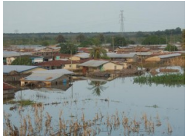
Flooded houses in one of the most affected districts in the Eastern Region/GRCS
