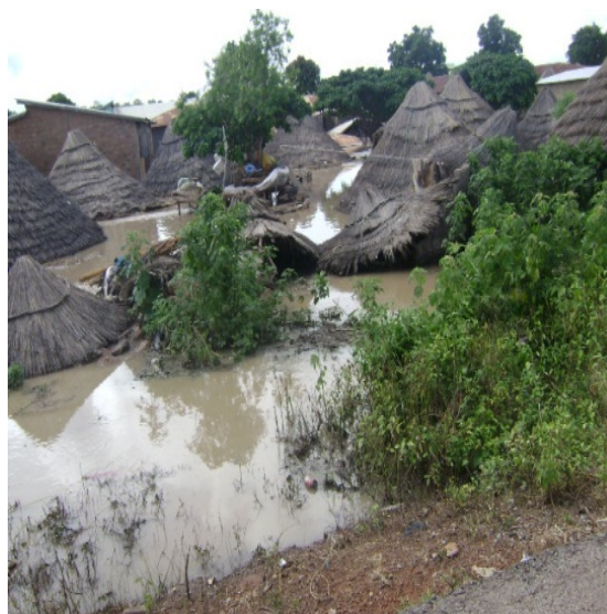
Flood at Siguiri/ Kéniébakoura during the assessment by Red Cross volunteers Photo: Red Cross of Guinea
