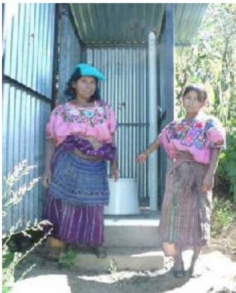
GRC volunteers helped build latrines for 64 families in Patalup.
