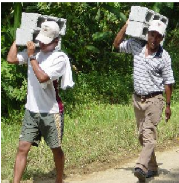
The water and sanitation project carried out in the Darién provided five communities with a safe, 24-hour water source.
