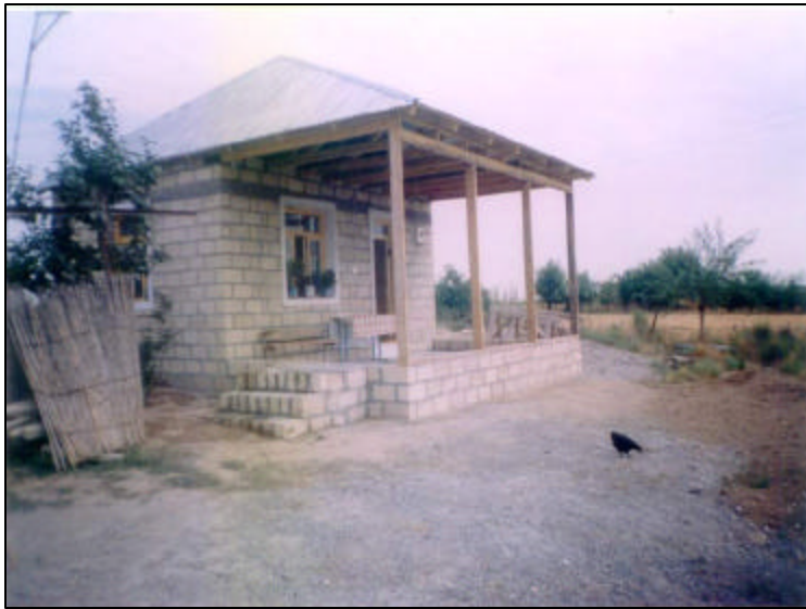
Rebuilding life: the Federation helped 830 returnees reconstruct their homes in Alkhanli and start again after years of displacement.
