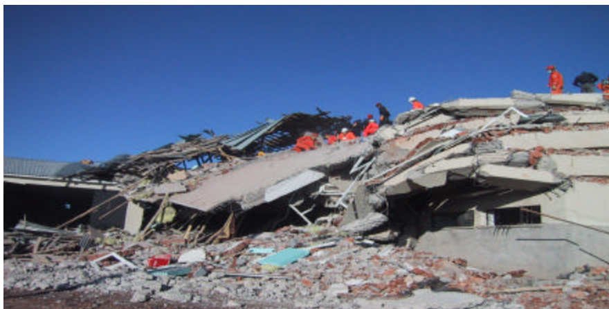
Destruction: over 170 people died in the Bingol earthquake.
