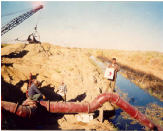
Drainage mitigation project in Turkmenistan, Mary province
