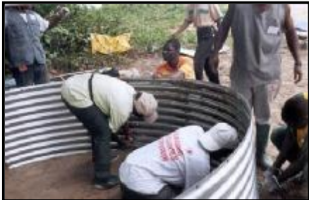
Tank construction in progress
