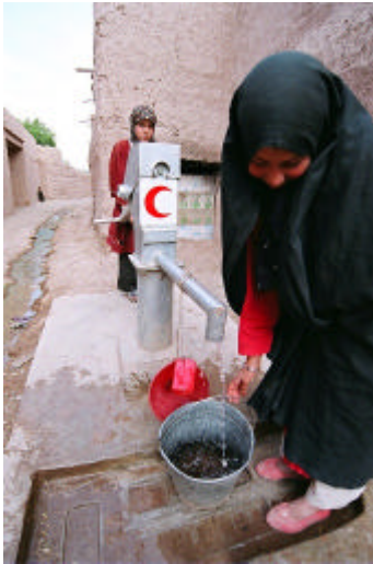
Red Crescent community constructed wells benefit thousands of people
