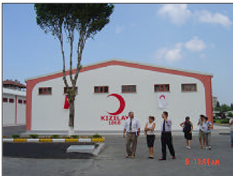
Turkish Red Crescent regional disaster response and logistics centre in Istanbul
