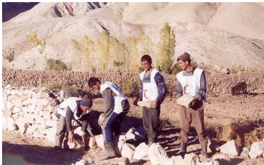
LDC members clean the mud stream ways to protect the village against mudflows
