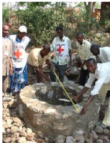
Red Cross Volunteers rehabilitating the same well.
