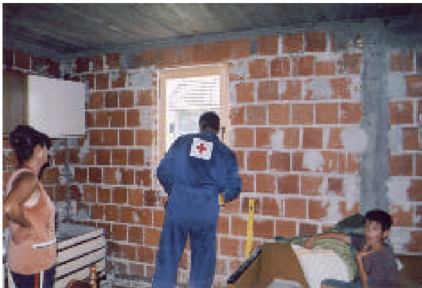
RCSBiH has worked in the community to make homes secure
