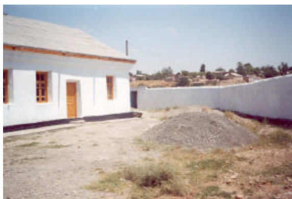
The Ganchi district branch office after the renovation
