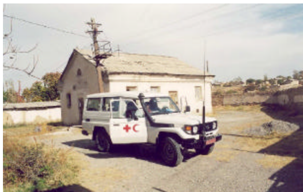
The Ganchi district branch office before the renovation
