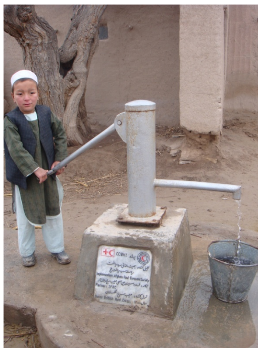
A young child is using the newly constructed well as a safe drinking water source in Shortepa district of Balkh province, northern Afghanistan. Photo: International Federation
