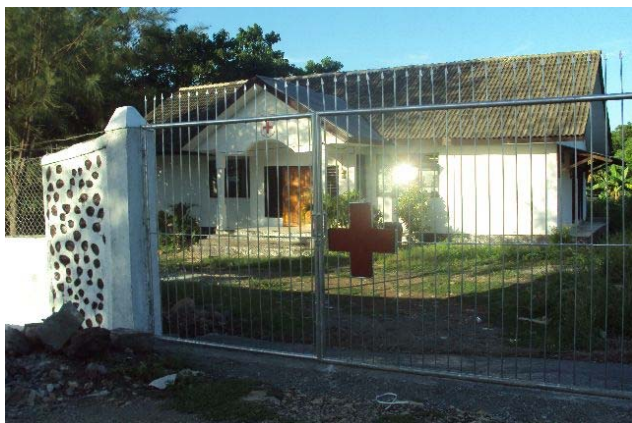
The Suai branch building rehabilitated with its new fence built by volunteers. Photo: AVI volunteer
