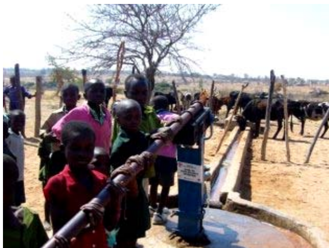
Maneta Primary School in Buhera District in Manicaland Province, where 450 students and 200 families in the area are benefiting from this borehole.
