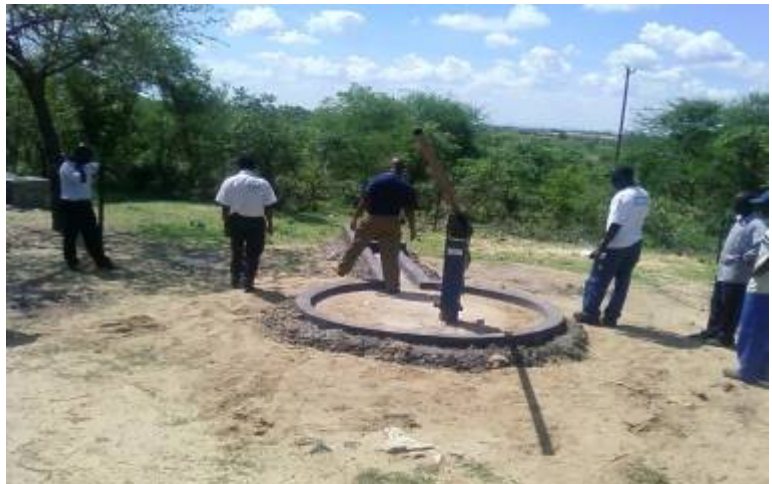
Completed rehabilitated borehole at Nyamuyaruka village in Mudzi district, Mashonaland East
