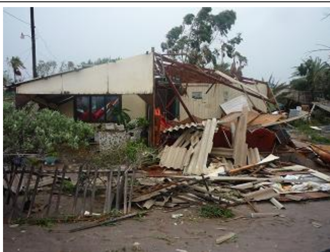
An affected house in Baja California. Source: Mexican Red Cross
