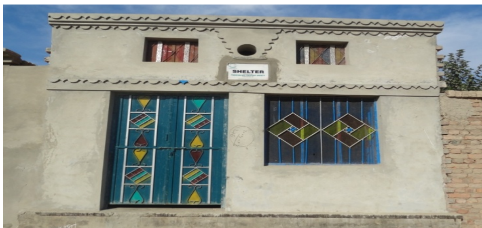
Completed shelter in Muzaffargarh, Punjab. Photo: IFRC
