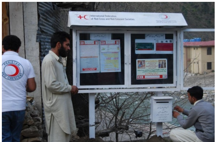
Installation of the beneficiary community notice board in KP. Photo: PRCS
