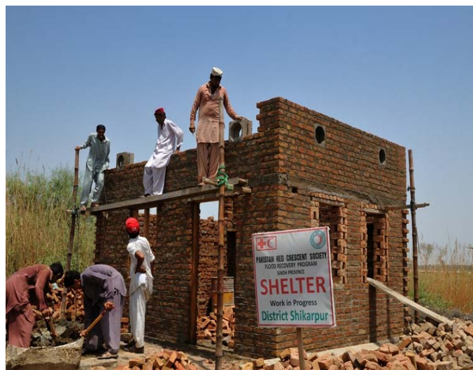
Shelter construction in progress, Shikarpur District, Sindh province. Photo: IFRC
