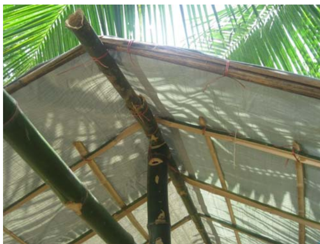
People used local bamboos and ropes to prepare their emergency sheltering in Cox's Bazar district. Photo: IFRC.
