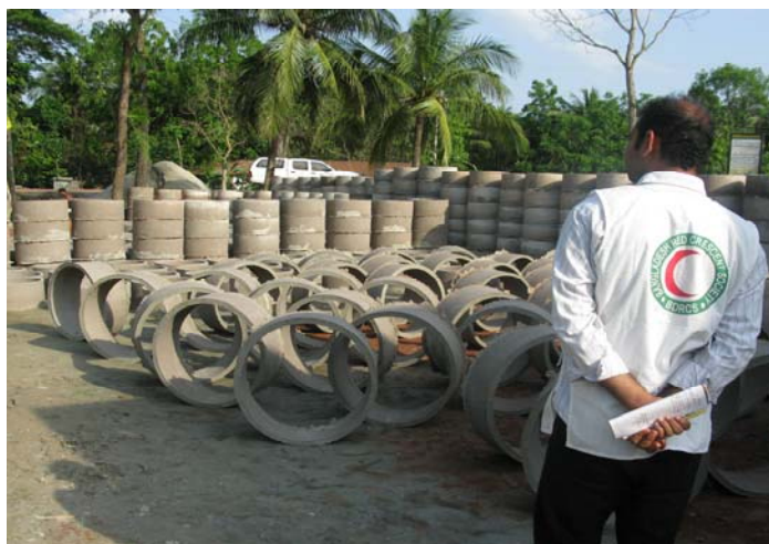
Red Crescent volunteers involved in supervision and monitoring of household latrine materials construction in Satkhira district. Photo: BDRCS.
