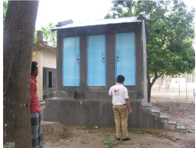
BDRCS/IFRC has constructed five latrines, in each community, which contained one bathing chamber and two latrine chambers. Photo: IFRC.
