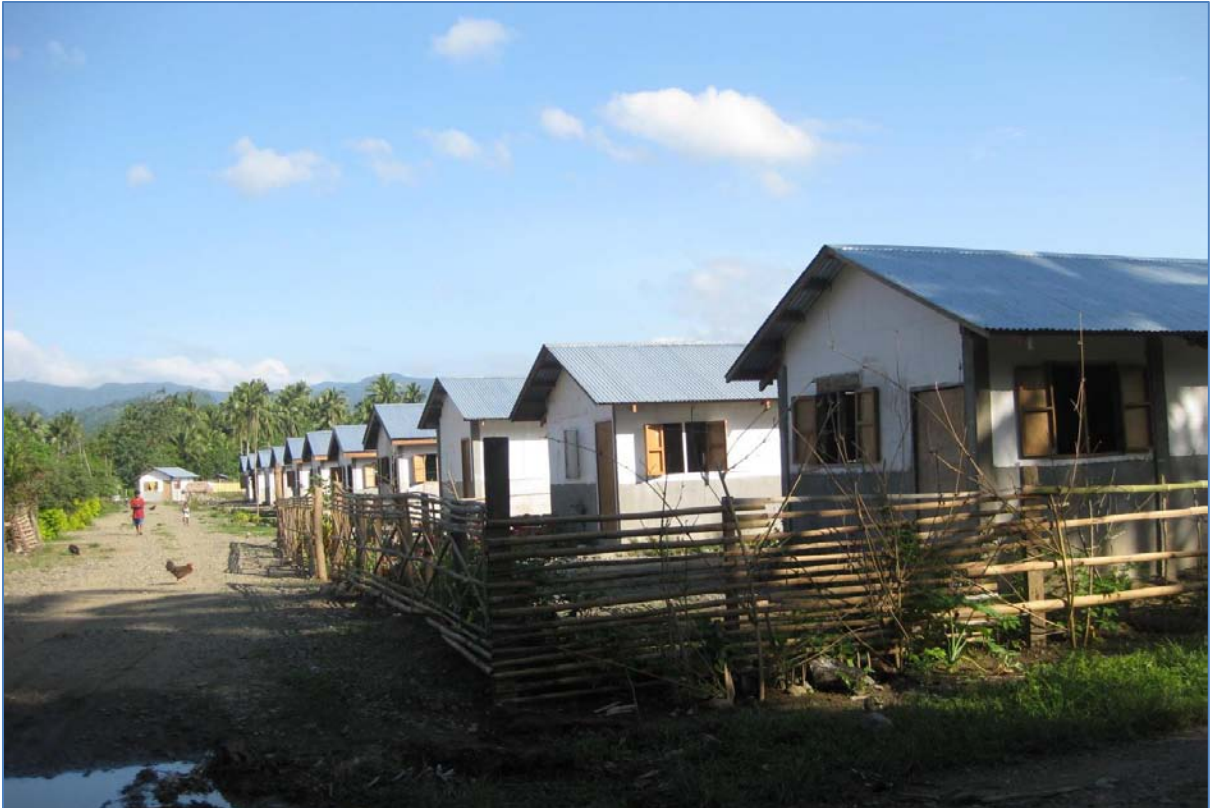
A total of 170 families (100 in Aurora, 43 in Ifugao and 27 in Quirino) were assisted and rebuilt typhoon-resilient shelter with latrines. Photo: Philippine Red Cross
