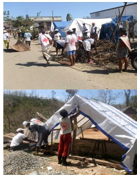
Volunteers assisting in construction of temporary shelters Brickaville/Photo MRCS
