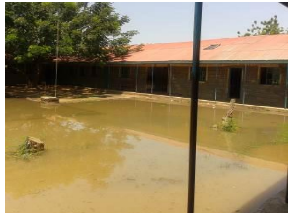
Salabani Primary School engulfed by water from Lake Baringo. Photo/KRCS.
