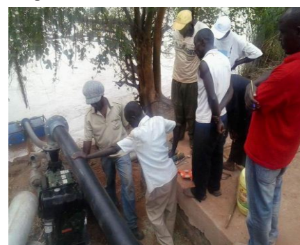
Rehabilitated irrigation pump machine. Photo/KRCS.
