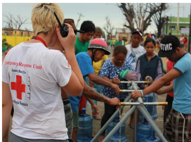
Spanish Red Cross water and sanitation M15 ERU operational in Tolosa, Leyte, about 30km south of Tacloban City. Photo: Spanish Red Cross
