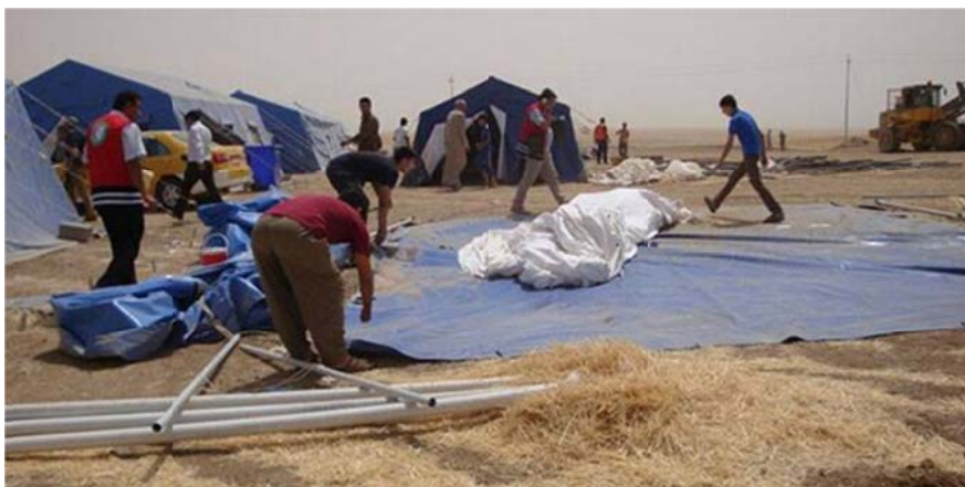
Iraqi Red Crescent response teams erecting emergency shelters to accommodate the displaced families from Mousl. Photo: IRCS
