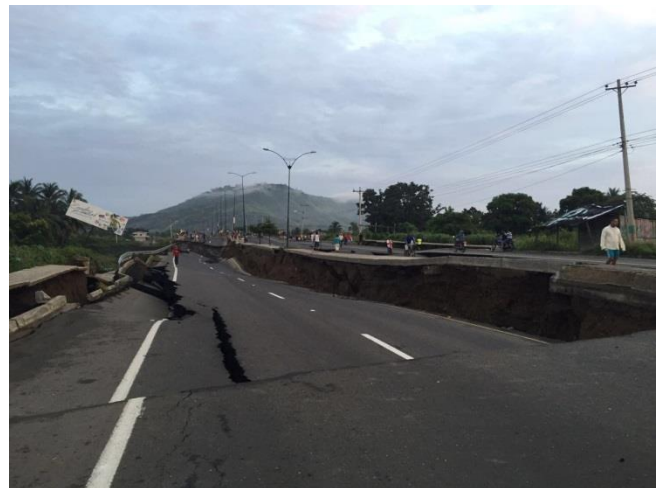
Collapsed road in an affected area. Source: Ecuadorian Red Cross
