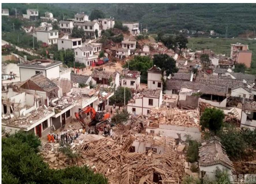
Collapsed houses in affected areas. Photo by media163.com.
