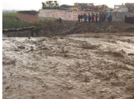
Minor floods in Arequipa province delayed construction works.
