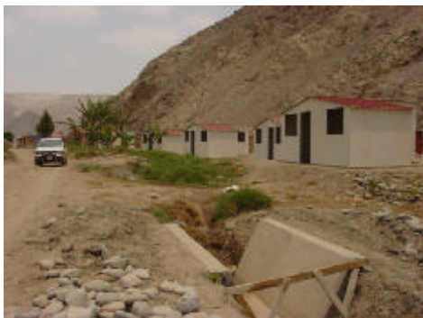
Completing 33 housing units in Tambo Valley (Arequipa).
